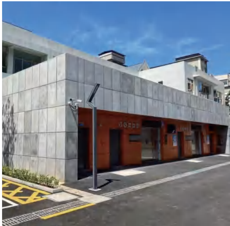
GAOSHAN STREET INTELLIGENT PARK- ING BUILDING
