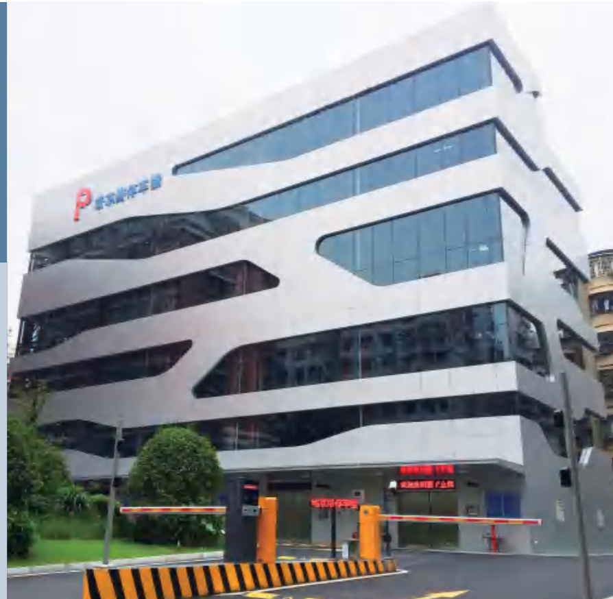
RUIJING ROAD STEREO PARKING BUILDING
