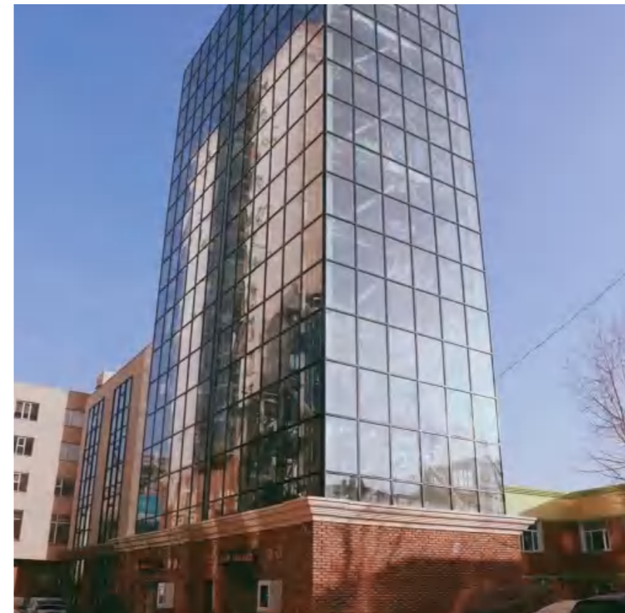
Mongolia Orchlon Twin tower project
